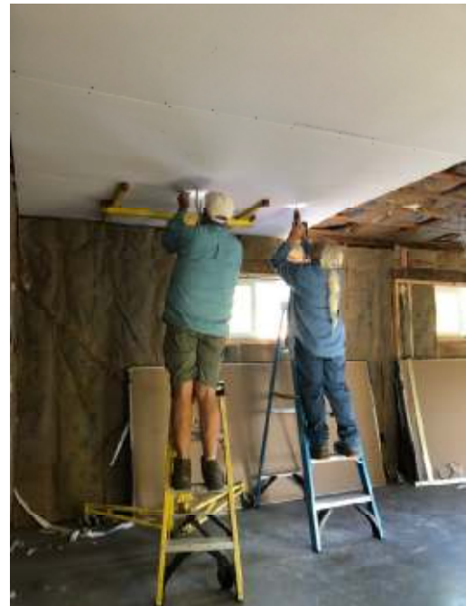
Kurt and Sonny worked during Harvest Fest weekend to put up sheetrock in the Junior Grange Hall.
