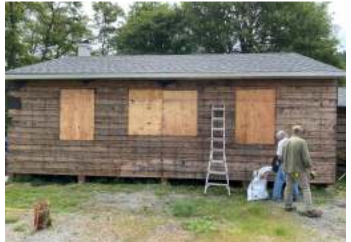
MRG Junior Hall, stripped to be remodeled this summer.
