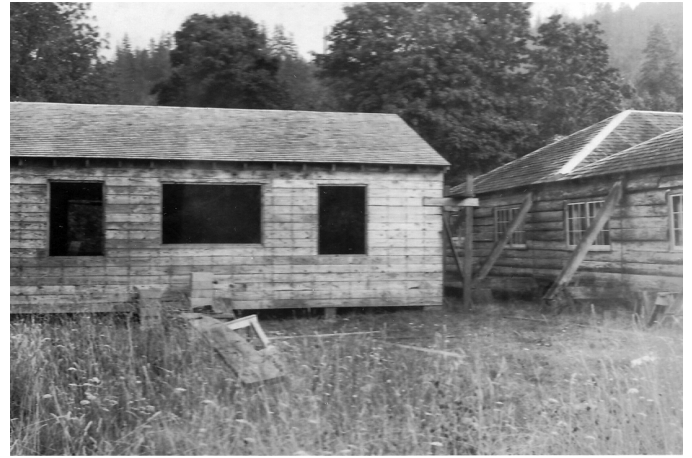
1955, Marys River Juvenile Grange Hall under construction.
